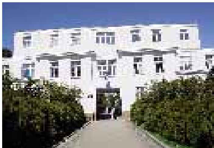
The building of the former “Franko Lisica” military barracks in Zadar that will be the future premises of the European Centre for Cross-Sectoral Cooperation.
